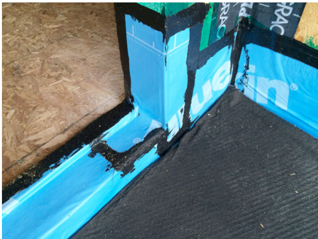
Photograph 5: Drainage Matt —Membrane waterproofing is stripped into the pan flashed balcony door opening. Note the drainage mat installed over the top of the membrane waterproofing. Also note the mastic application sealing the vertical portion of the balcony deck waterproofing membrane to the wall sheathing.
